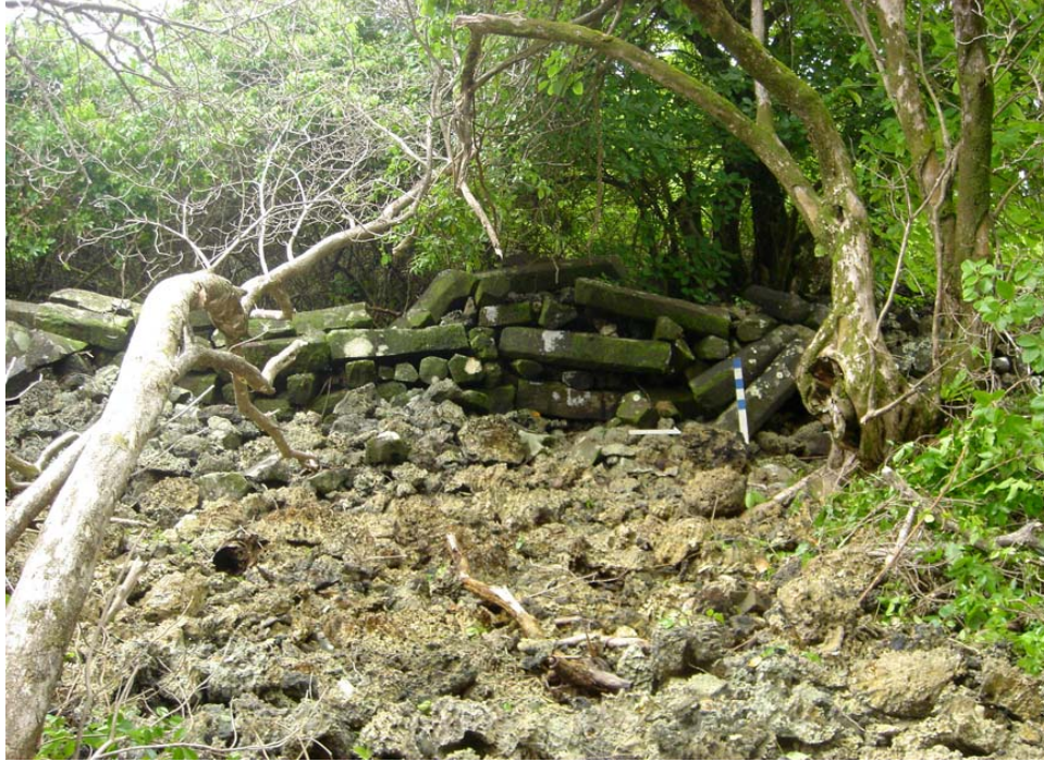
Figure III-14. East end of the lolong forming the main part of Sapwuhtik B Islet, Nan Madol (PoC3-1) is shown here after clearing. This structure, Feature SWUB-1, consists of an enclosing wall made with basalt columns on top of coral rubble fill and a central main tomb feature. [photo nm00456; k. seikel].
